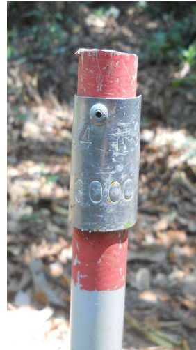
Figure 3: Example of a picket tag showing the trail name and distance along the trail (3000m).
